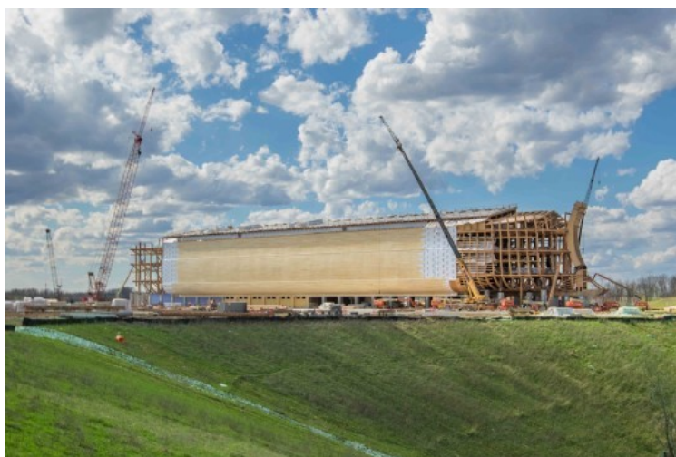
Ark Encounter under construction
